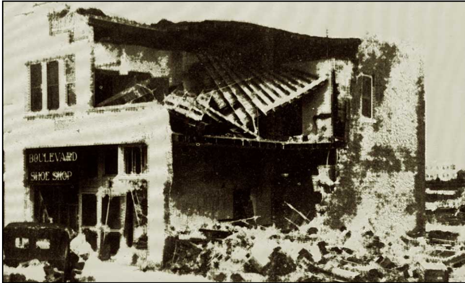
Figure 2-6 Building damage from 1926 hurricane, Miami, Florida.
