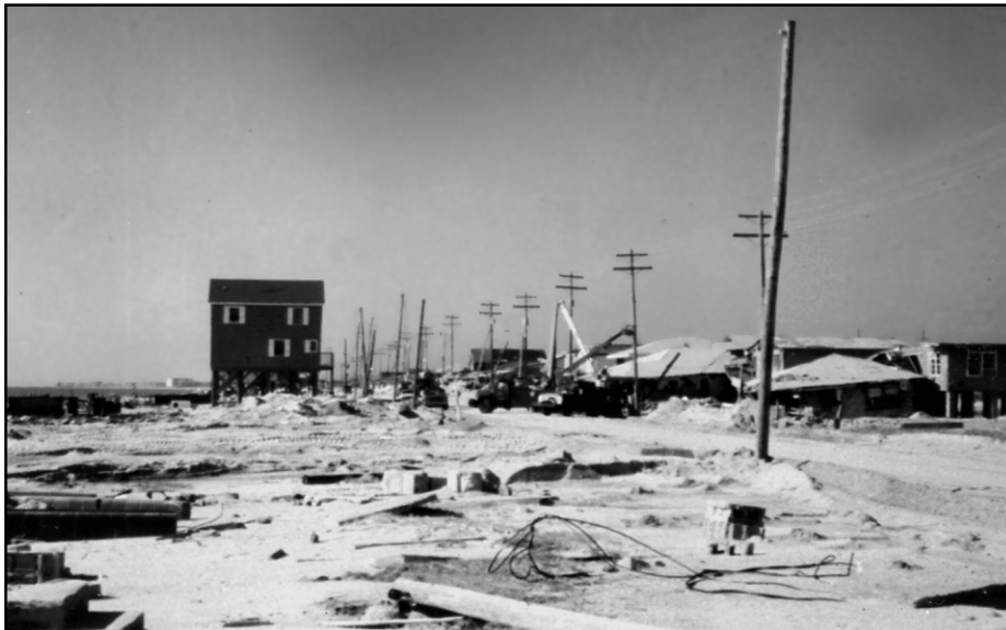
Figure 2-11 Hurricane Hugo (1989), Garden City Beach, South Carolina. House on pilings survived while others did not.
