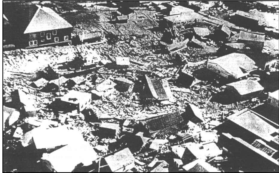
Figure 2-22 1964 Good Friday earthquake. Damage in Kodiak City, Alaska, caused by the tsunami of the 1964 Alaskan earthquake (from Wilson and Tørum 1968).
