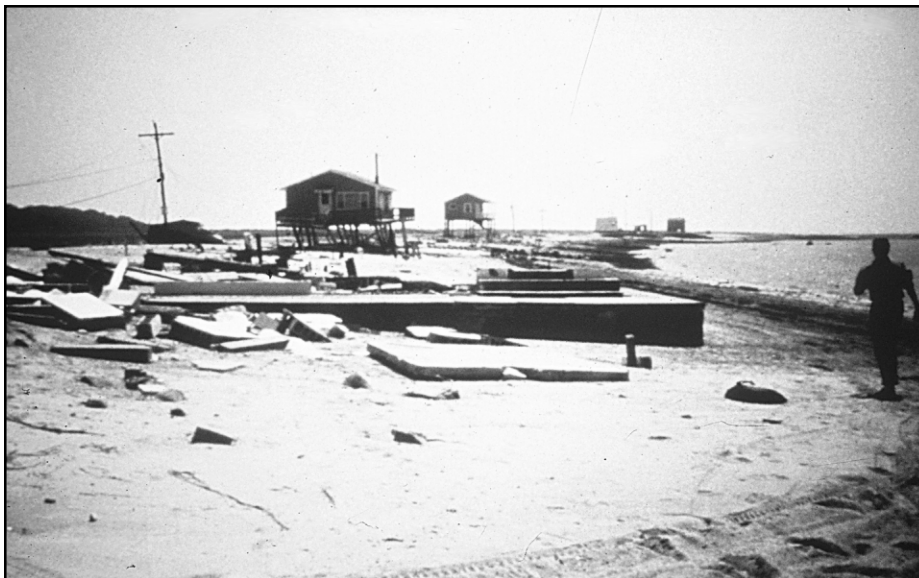
Figure 2-3 Hurricane Bob (1991) destroyed 29 homes along this reach of Mattapoisett, Massachusetts. Photograph by Jim O'Connell.
