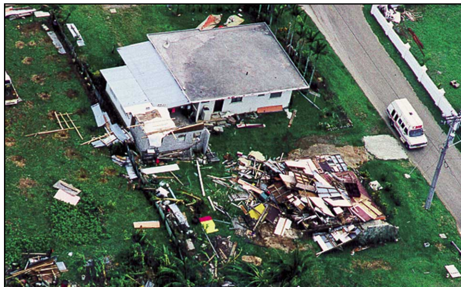
Figure 2-26 Typhoon Paka (1997). Although damaged by the storm, the concrete house in the upper part of the photograph survived, while the wood-frame house next to it was destroyed.
